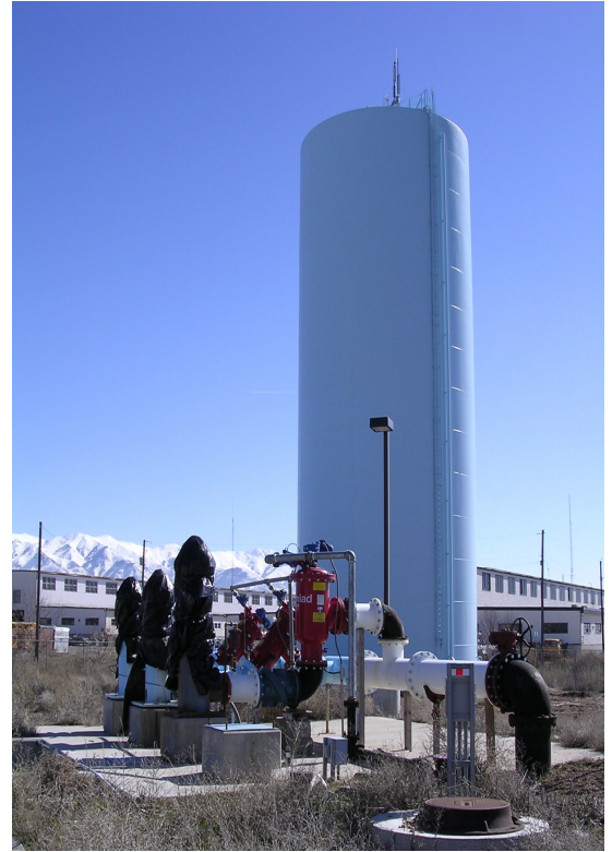
Syracuse City's Storage Facility
